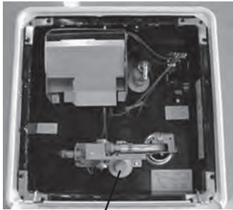
Water Heater Drain Plug
